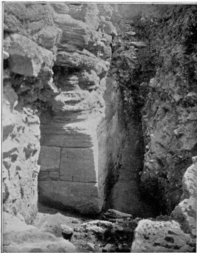
**Fig. 12.16** Wall at Hissarlık, showing contrast between weathered and protected courses (From Butler 1922: 216a. By permission of the Master and Fellows of St John's College, Cambridge)
