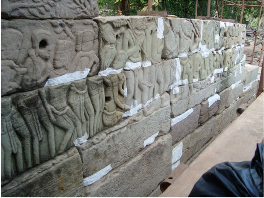
Fig. 9 Dismantling of bas relief in the SE sector, preconsolidation prior to removal (Global Heritage Fund)
