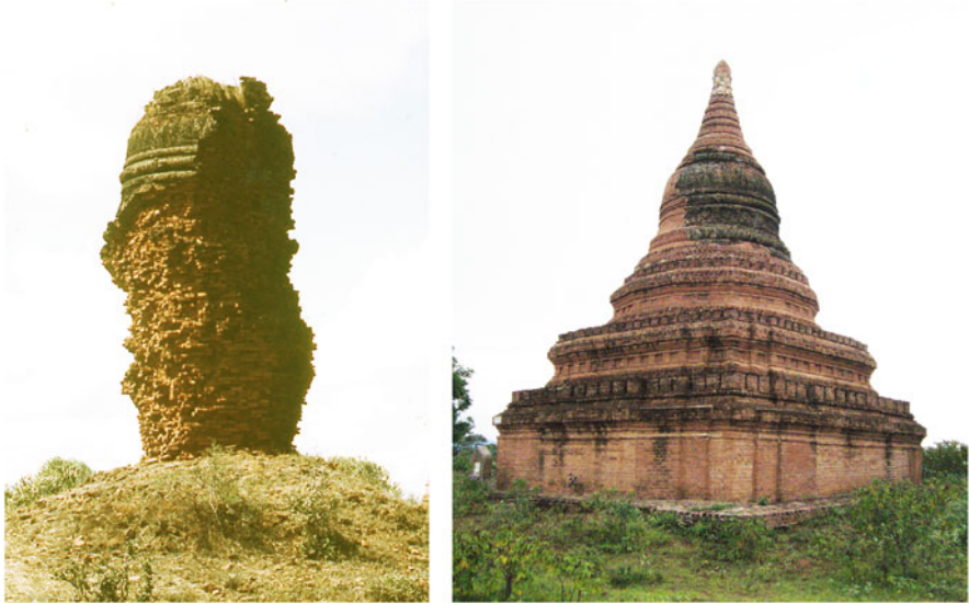
Fig. 5 Stupa 770, Pagan. Left : Condition in 1987 (Pichard 1987); Right : In 2006 after beautification. In this case, the reconstruction of missing parts has certainly prevented a future collapse of the monument. The details and proportions of the reconstructed parts are, of course, conjectural (Berliet 2006)
