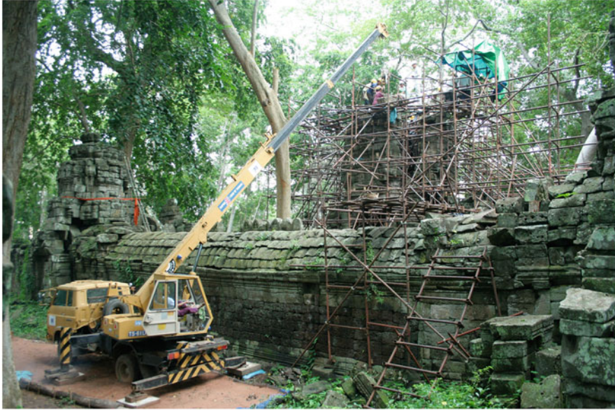
Fig. 11 Dismantling face tower 18N using a crane (Global Heritage Fund)
