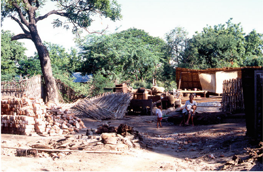
Fig. 3 June 1990. Ordered to demolish their own houses, the villagers of the walled city wait for army trucks to transport the materials to New Pagan. In compensation each family received one kilogram of nails to rebuild their homes (Pichard 1990)
